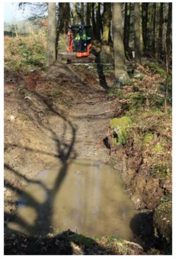
**Photo 15:** Looking northeast along the section of the leat just north of the northern bridge abutment after partial excavation by machine
