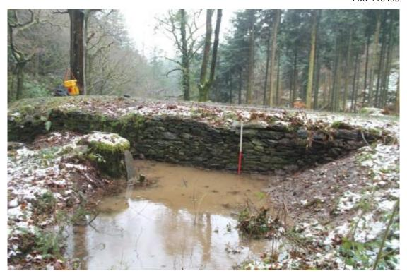
**Photo 9:** The northeast face of the northern bridge abutment after moss removal and after excavation of the leat, with a 1m scale
