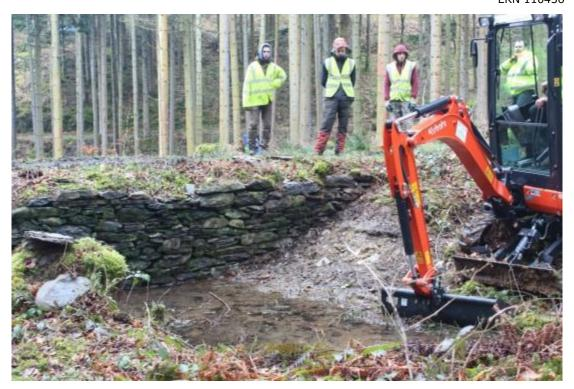
**Photo 12:** Excavation of the alluvial deposits in the leat by machine, facing west-southwest
