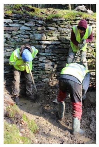
Photo 20: Excavating the leat southwest of the bridge abutment by hand
