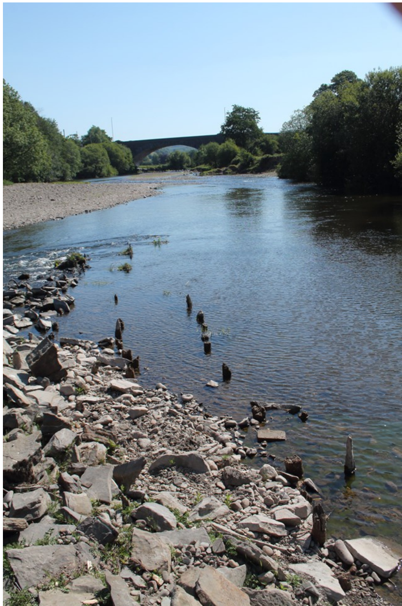
Weir downstream of Llandeilo Bridge
