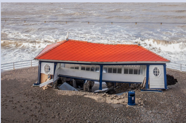
Bathrock Shelter, Aberystwyth, damaged by a storm in 2014.
