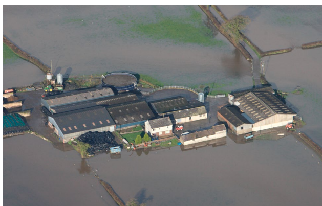
Glantowy Fawr farmhouse and farm on the floodplain of the River Tywi showing the effects of increased rainfall on historic assets.
