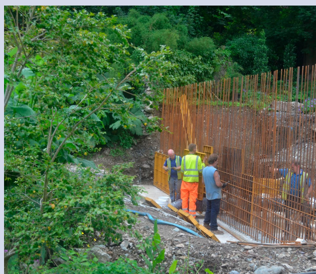
Adapted replacement stone wall at Plas Cadnant.
