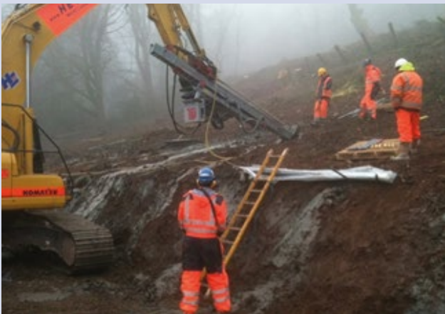
Repairs to the embankment near Llanfoist.
