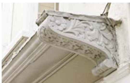
Far right: A fine shopfront, with classical detail, wrapped around the corner of Queen Street and Bridge Street (Crown Copyright; RCAHMW).
