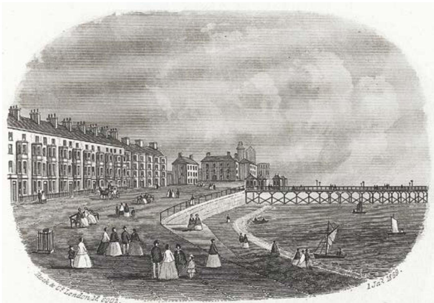
Above: Part of Marine Terrace and The Promenade, as depicted in 1867. The long terrace had recently been rebuilt: its predecessor was only two-storied (The National Library of Wales).
