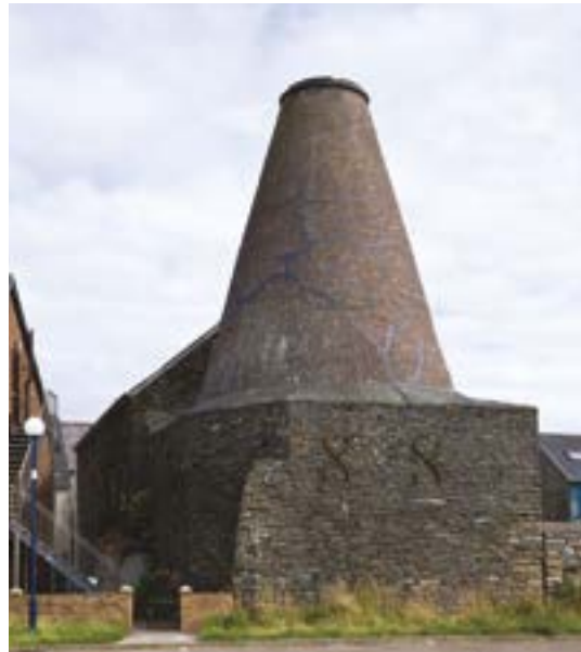
The former maltings is an important reminder of Trefechan's industrial past (Crown Copyright: RCAHMW).
