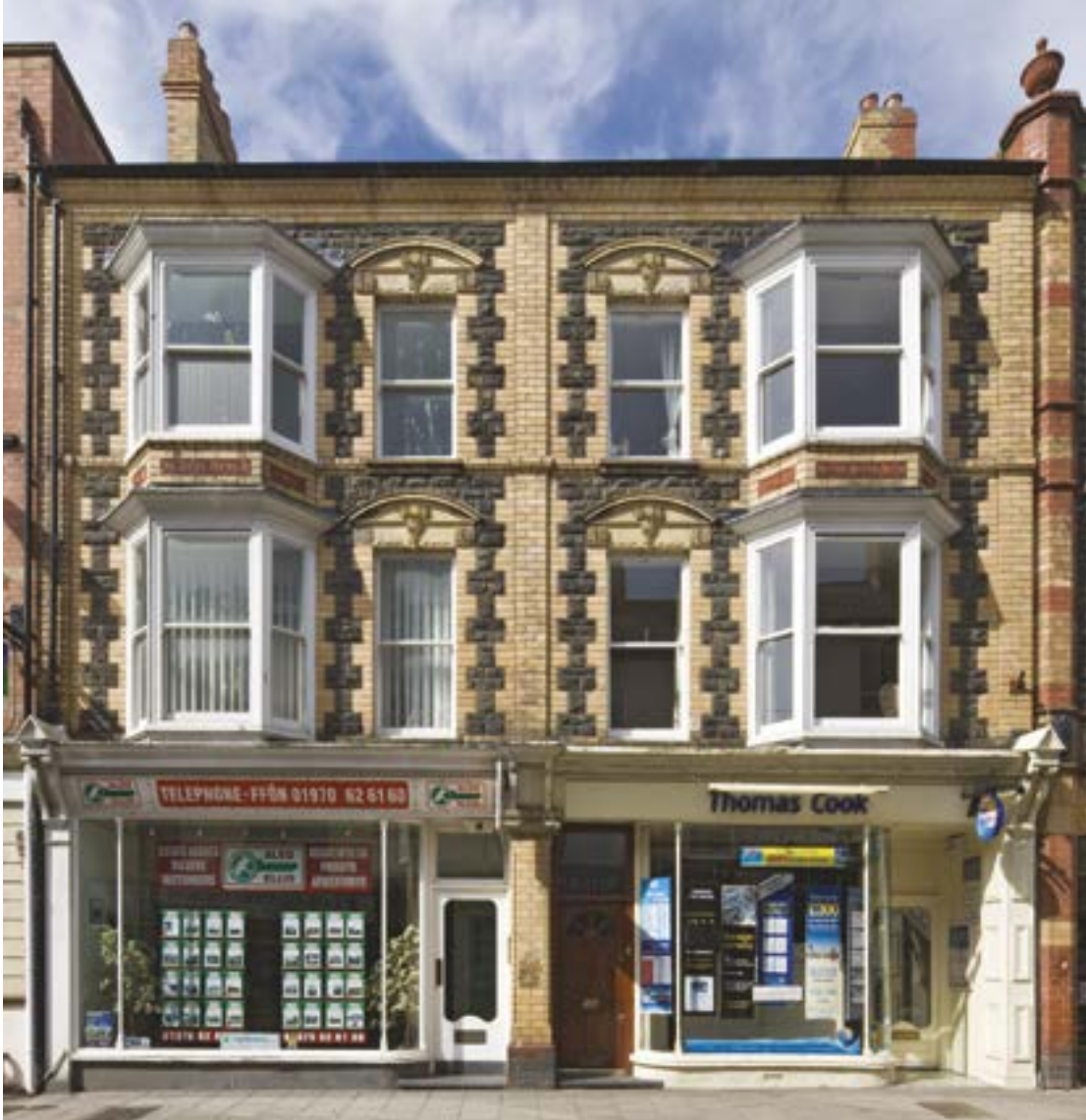
By the late nineteenth century, exposed stone was again used, often in combination with other materials and with a more pronounced dressing (Crown Copyright: RCAHMW).
