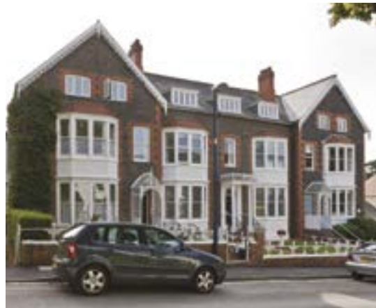
Left: Saint David's Road — large-scale terraced housing (Crown Copyright: RCAHMW).
