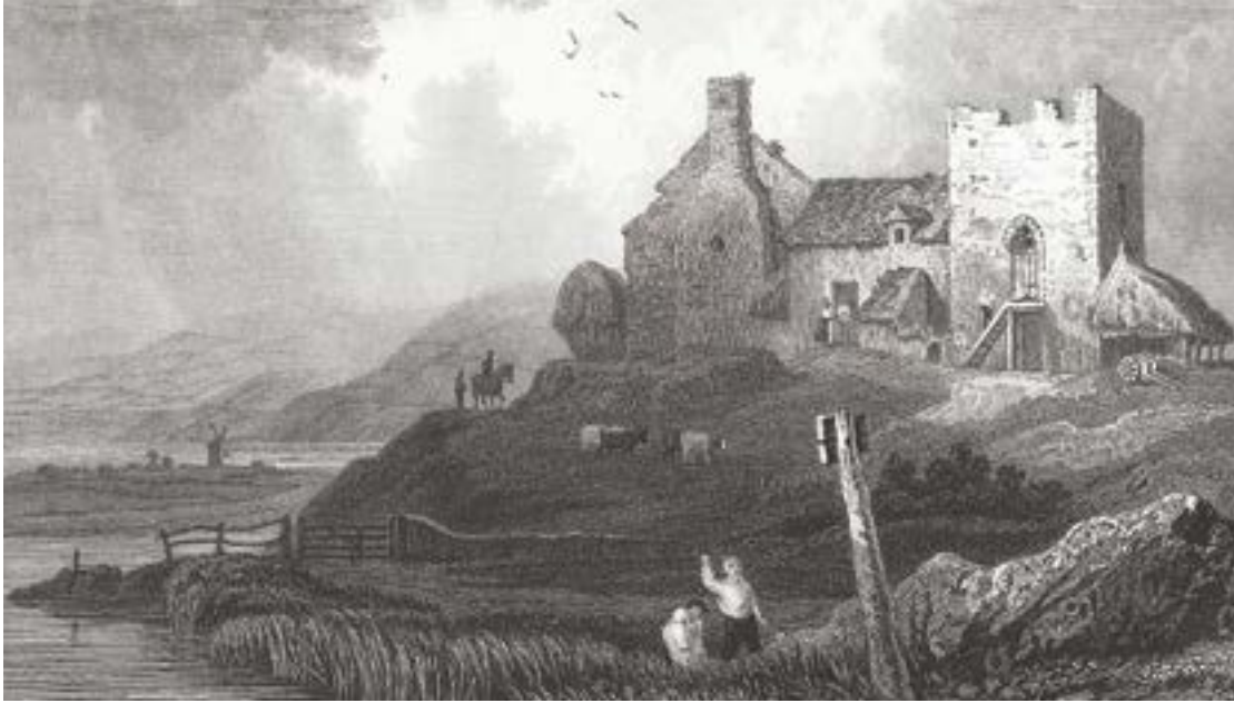
Left: Plas Crug, romantically assumed to incorporate a medieval castle, but probably an eighteenth-century folly (The National Library of Wales).
