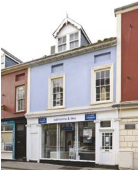
Far right: Stressed quoins and a rusticated lower storey with scribed render above, Saint Michael's Place (Crown Copyright: RCAHMW).
