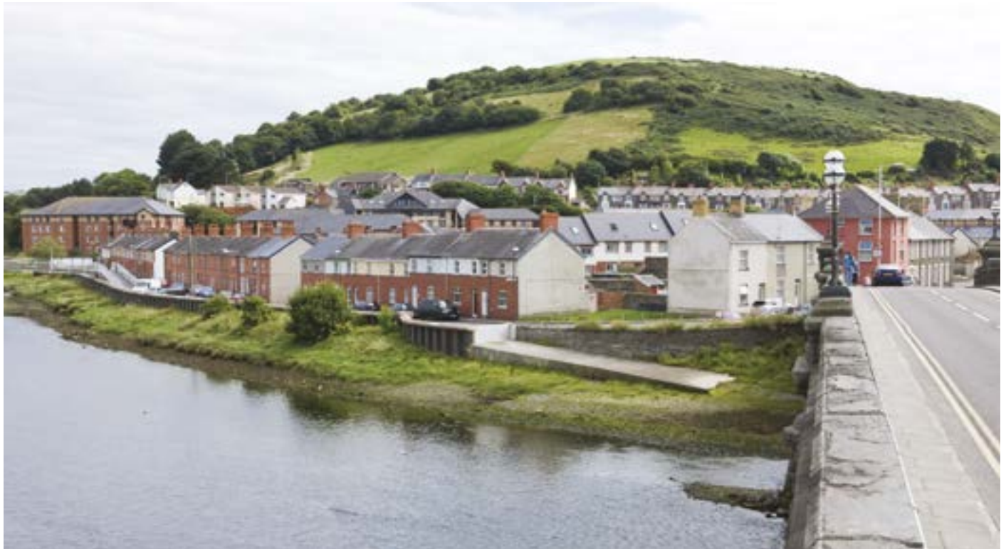
Early housing developments at Trefechan (Crown Copyright: RCAHMW).
