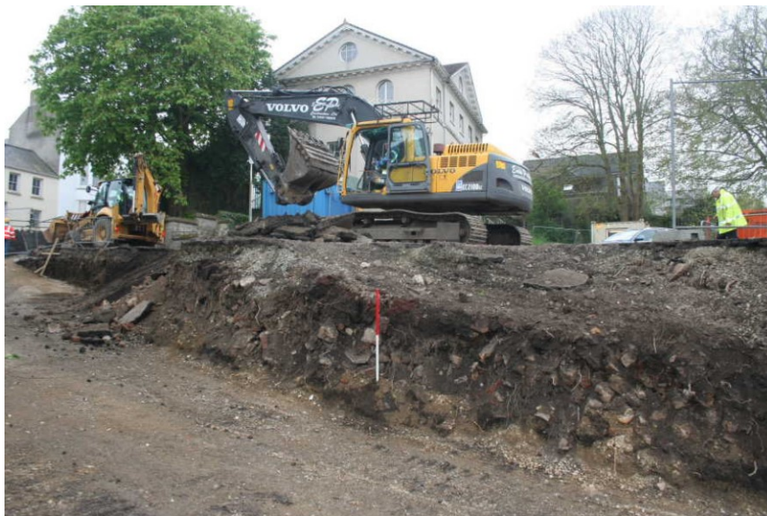
General shot showing the made ground on which Foley House (in background) and garden were established.
