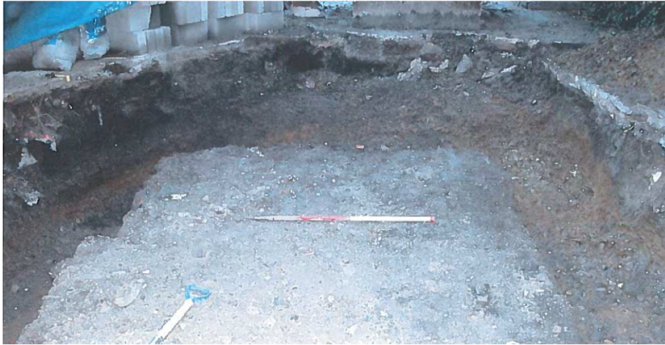
General view of the work at 1 Castle Terrace.
