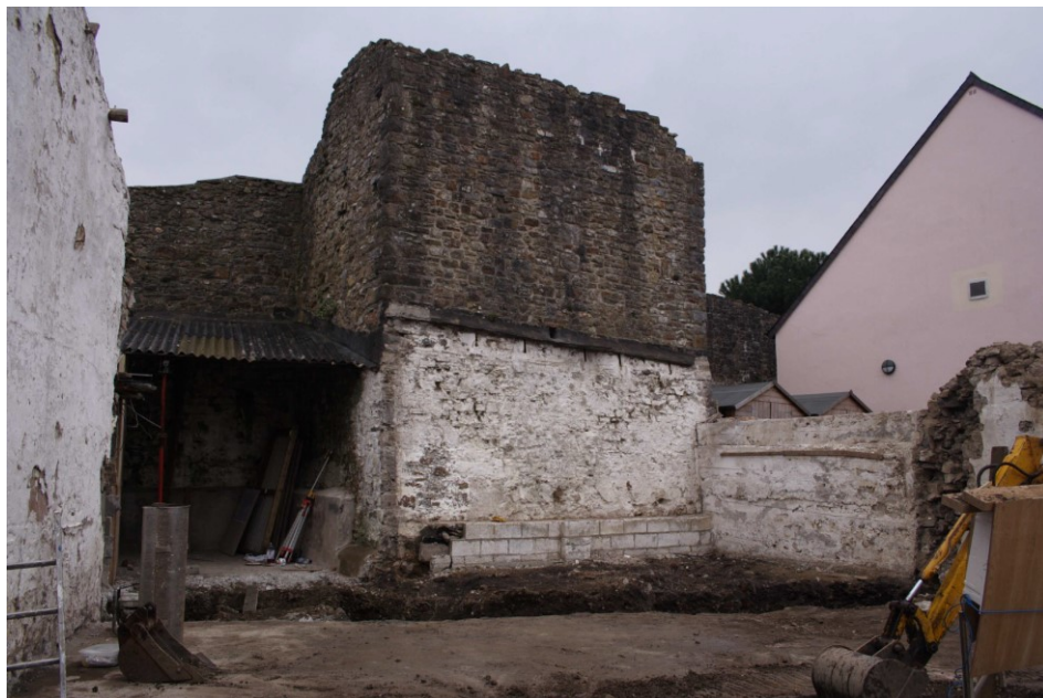
Photograph of the construction work in progress outside the castle walls.
