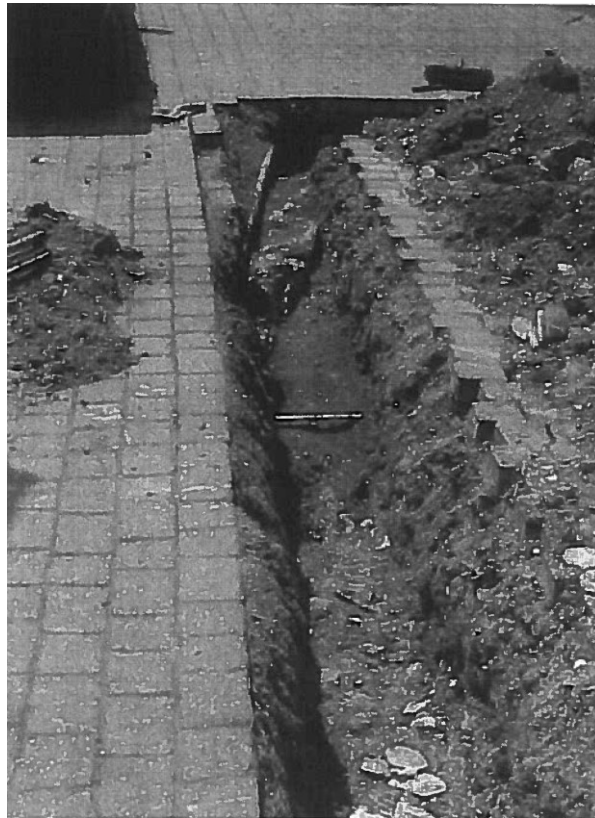
Wall foundations visible in the pipe trench to serve Tenby Museum.
