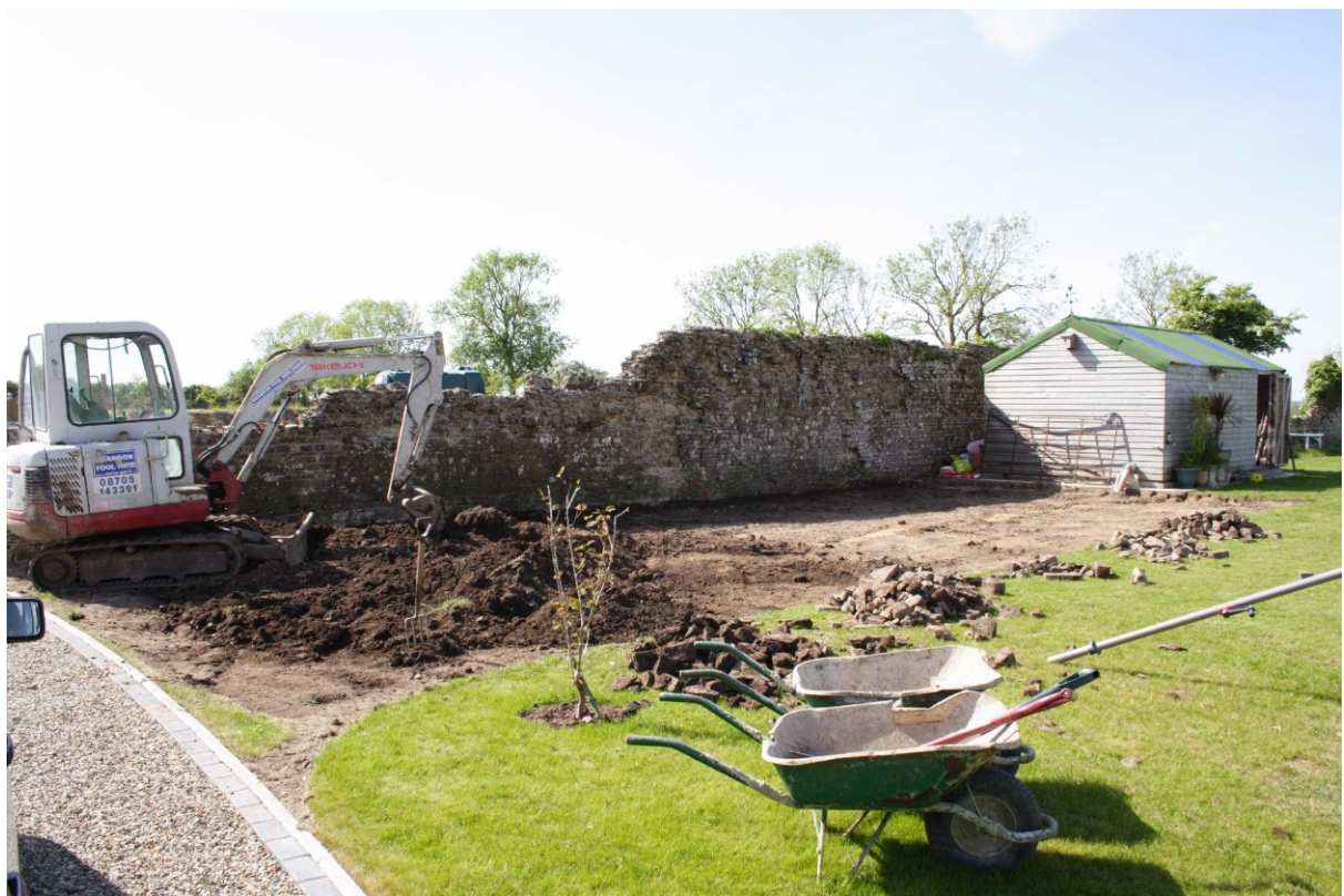
View of the topsoil strip during construction of a garage in the walled garden.
