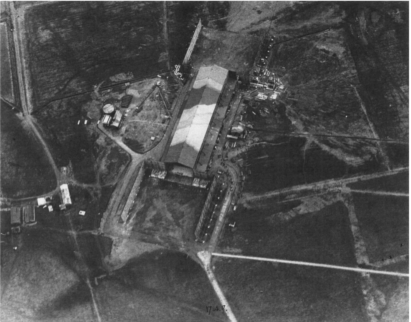
*View of RNAS Llangefni taken from an airship in 1917. Note the windshields at the ends of the shed and the gas plant to the left (Courtesy of Anglesey Archives).*
